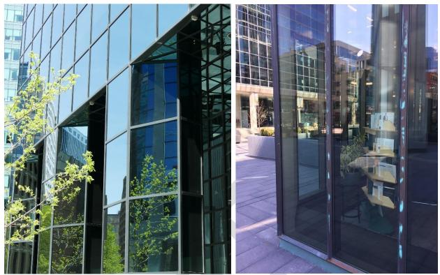
Figure 8: Potential design traps (mirror maze and black hole effect on left, corner glass on right).
